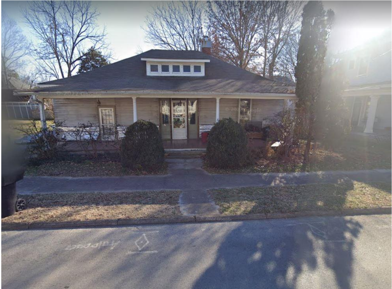
House in 2019- 444 East College
