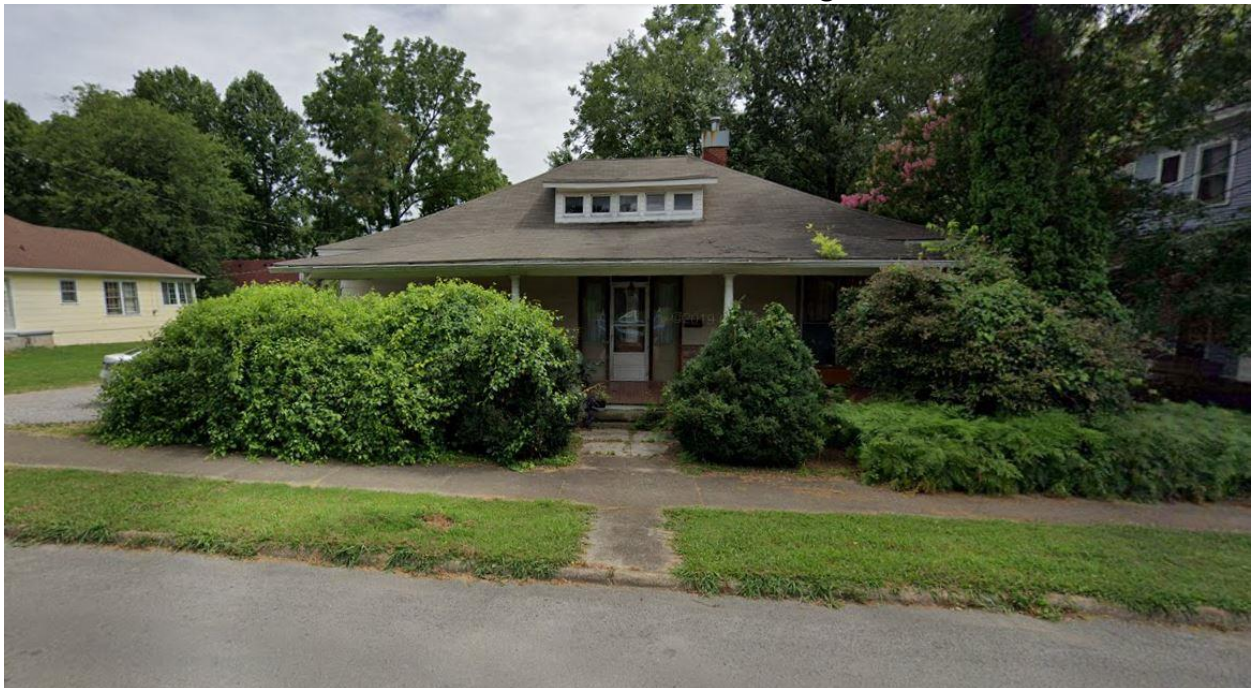
House in 2021- 444 East College
