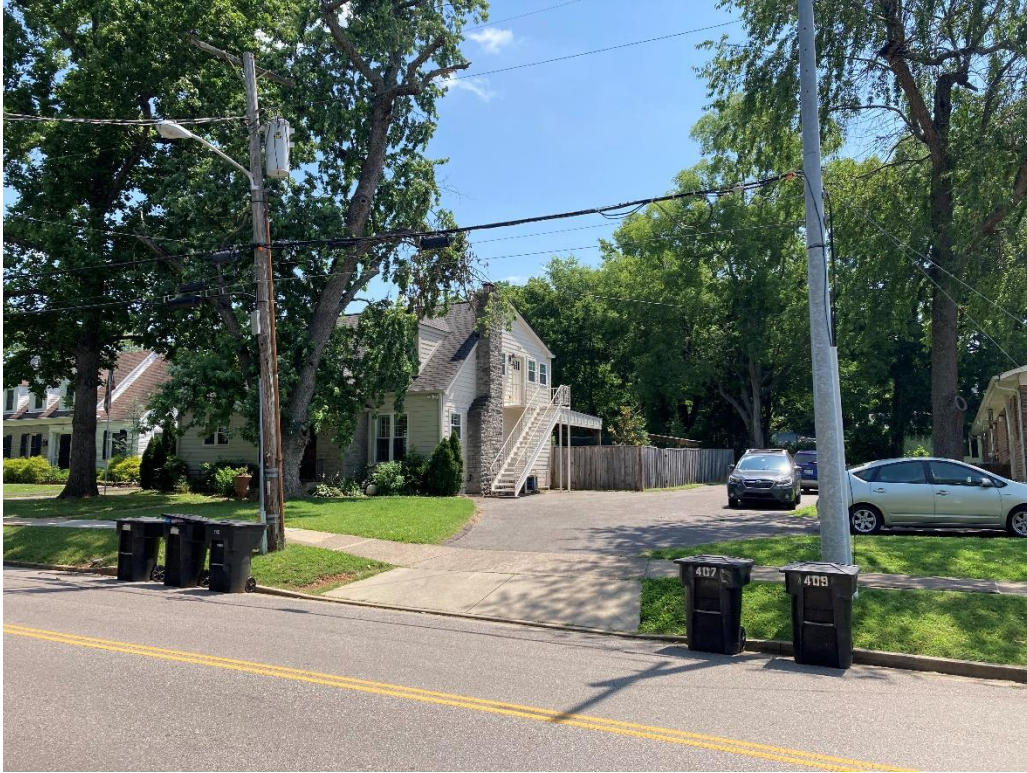
Existing House- 208 S. Maney
