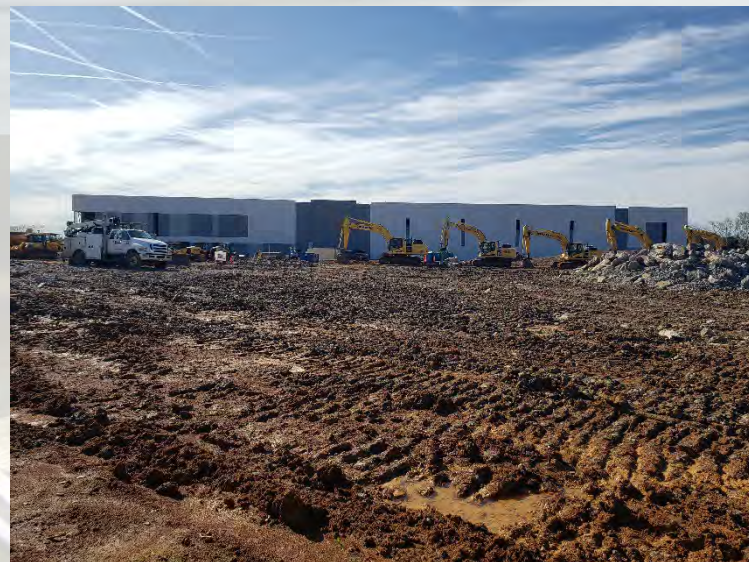
#6 (Existing construction on-site)
