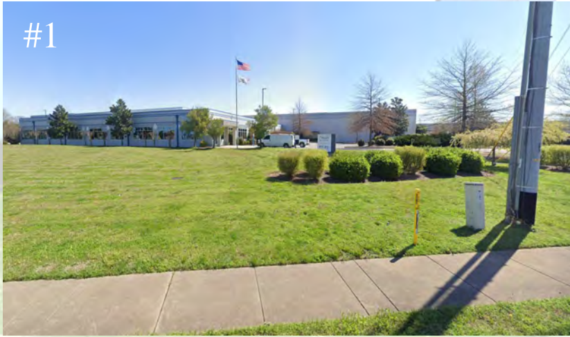
#1 The Perfect Equipment site is located to the northwest of the subject property.
