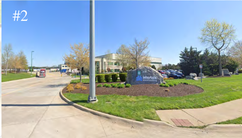
#2 The Interstate Warehousing site is located directly north of the subject property on the opposite side of Joe B Jackson Parkway.
