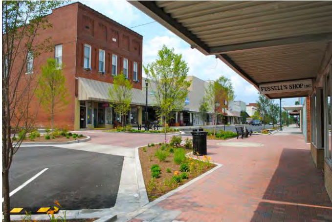
Raised crosswalk with chokers to reduce distance a pedestrian must cross the travel lane.
