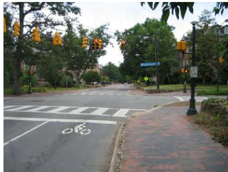
Pavement Marking indicating Bicycle Detector Loop Location
