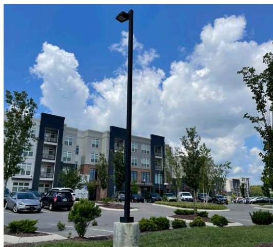
EXAMPLE OF STREET LIGHT
