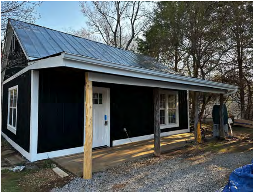
Front of Structure closest to Patriot Drive (South Side)
