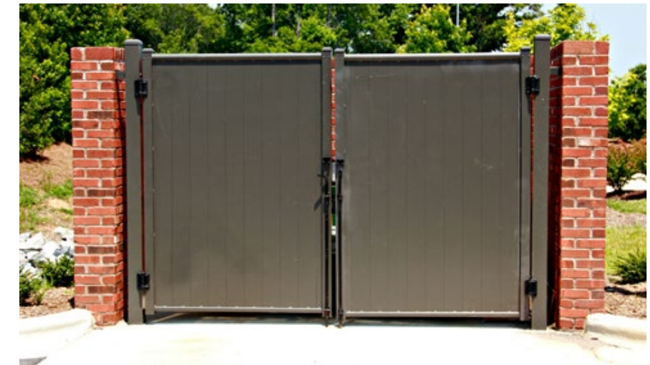
Example of Solid Waste Enclosure
