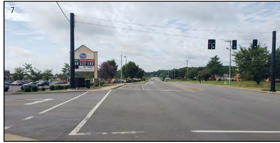
View of Kroger Shared Access Intersection Looking South
