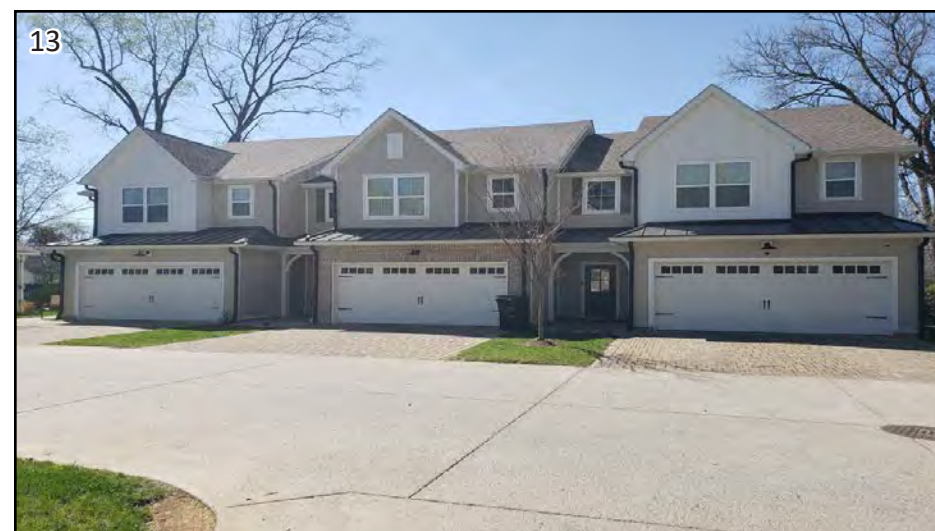
VIEW OF EXISTING REAR ELEVATION ON ADJACENT PROPERTY
