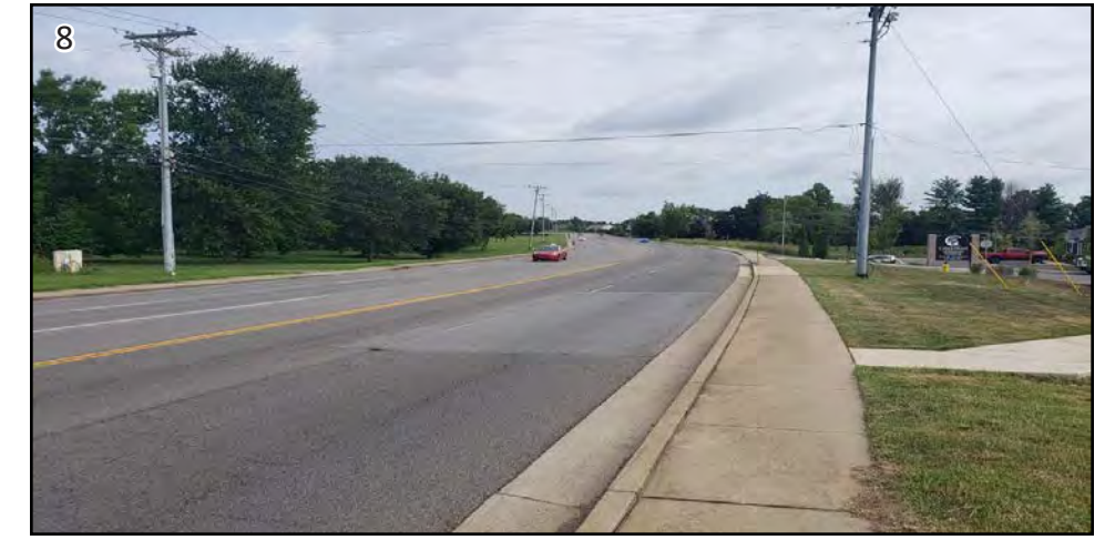
View from Existing Kroger Shared Access Intersection Looking North
