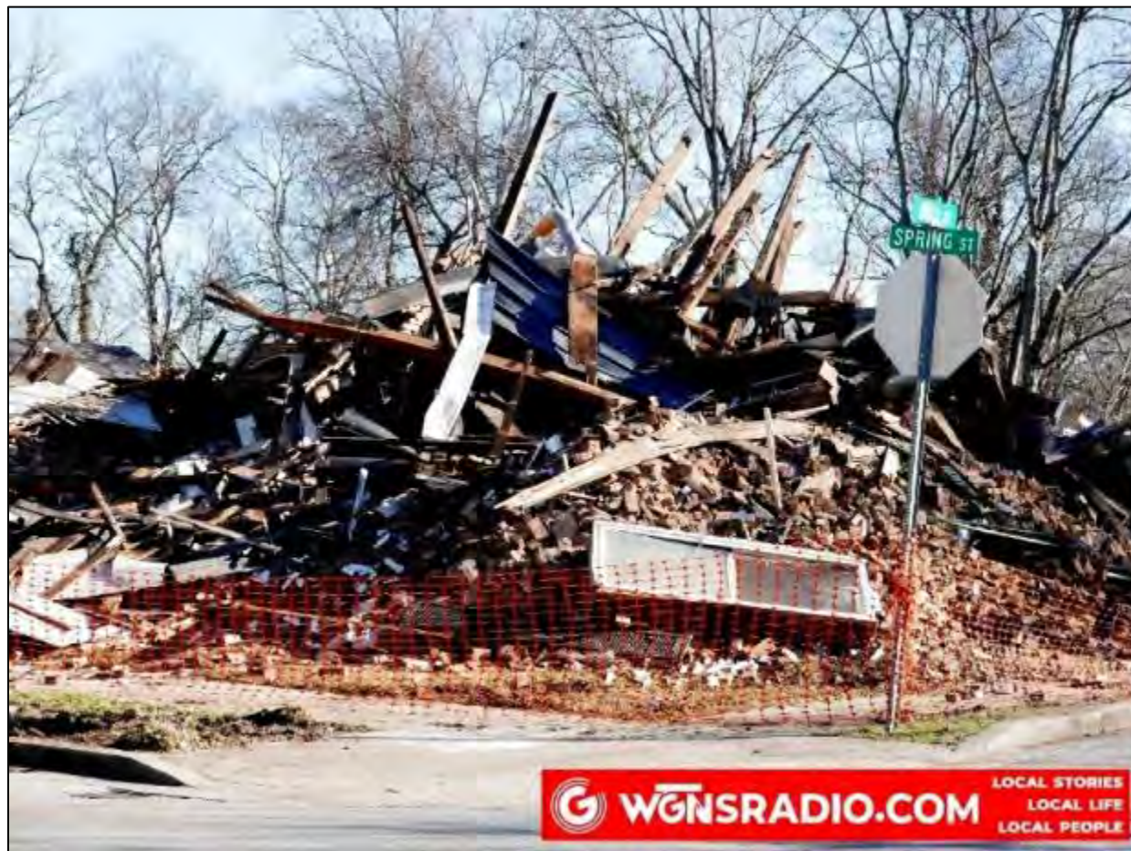
Figure 2: Demolition of the Collier-Lane-Crichlow House. From WGNSRadio, https://www.wgnsradio.com/article/78752/the-house-of-mayors-has-left-the-city .
