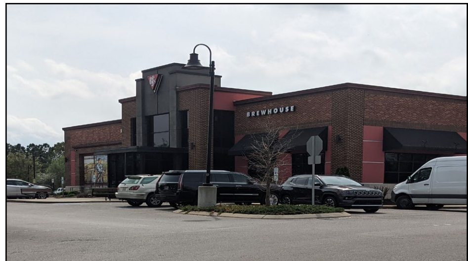
8 - Outparcel '8'- Currently Occupied by BJ's Restaurant & Brewhouse
