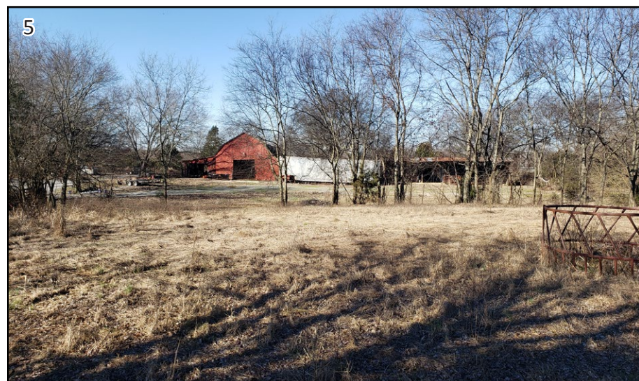
View of Existing Barn and Accessory Structures Looking West
