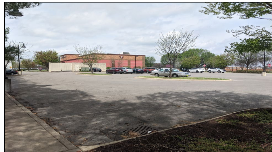
9 - Outparcel '8'- Currently Occupied by BJ's Restaurant & Brewhouse
