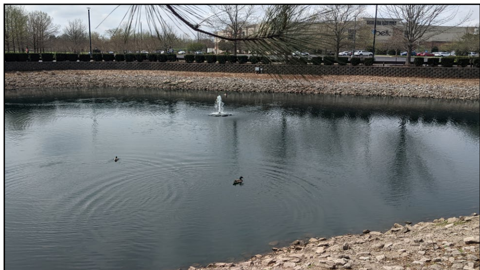
10 - Near Outparcel '8'- Stormwater Pond
