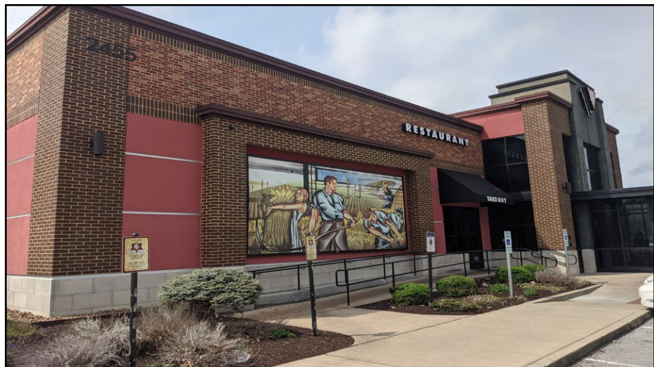
7 - Outparcel '8'- Currently Occupied by BJ's Restaurant & Brewhouse
