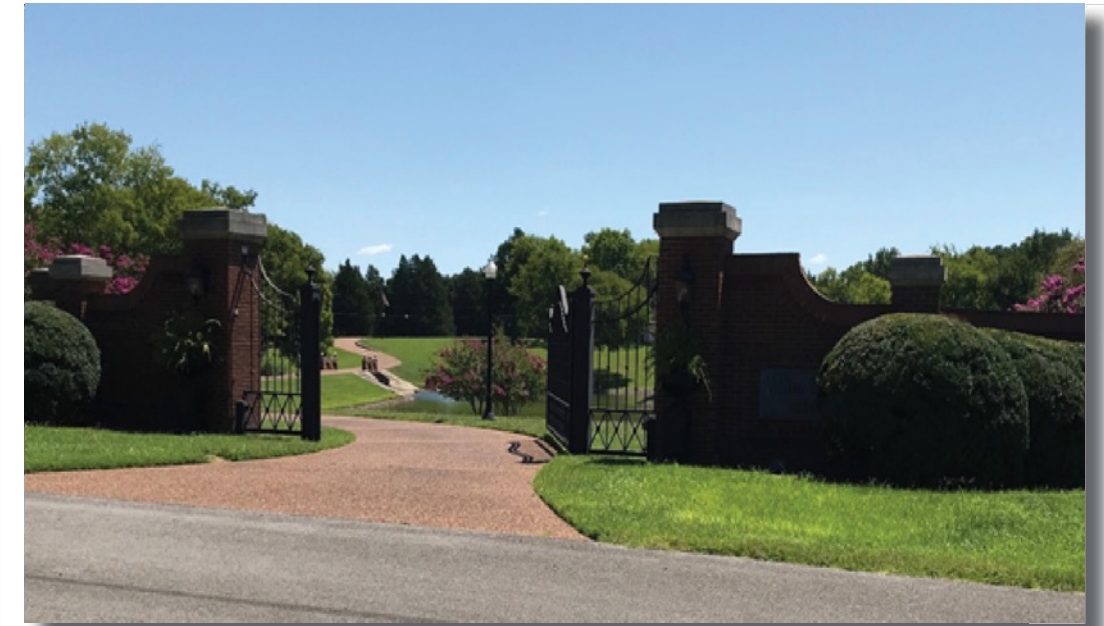
Existing northern entrance off of Racquet Club Drive
