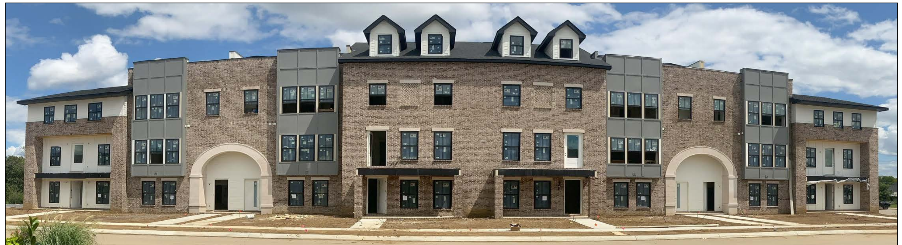
Front view of built units
