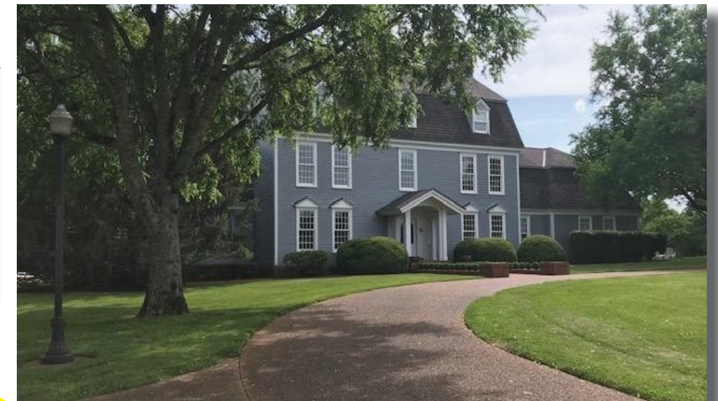
Existing Residence (To be converted to future club house)
