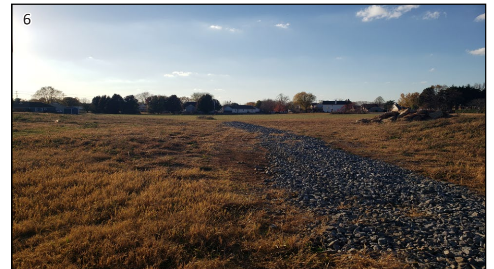
View From Southgate Boulevard Looking West
