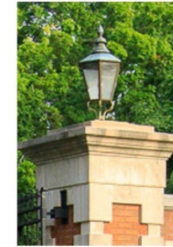
EXISTING GAS LAMP FIXTURE - ADAMS PLACE
