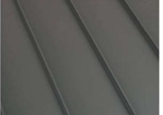
STANDING SEAM ROOF ACCENTS - MATCH EXISTING CAMPUS
