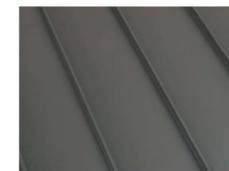
STANDING SEAM ROOF ACCENTS - MATCH EXISTING CAMPUS
