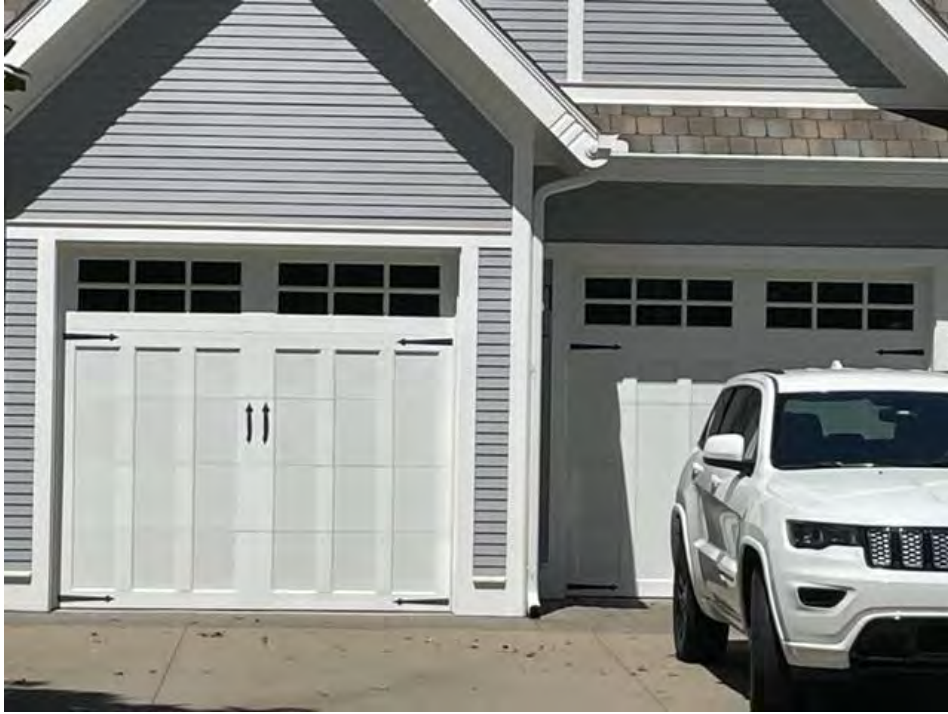
- wood clad metal garage door Steel door with 5/8" overlay 2017
