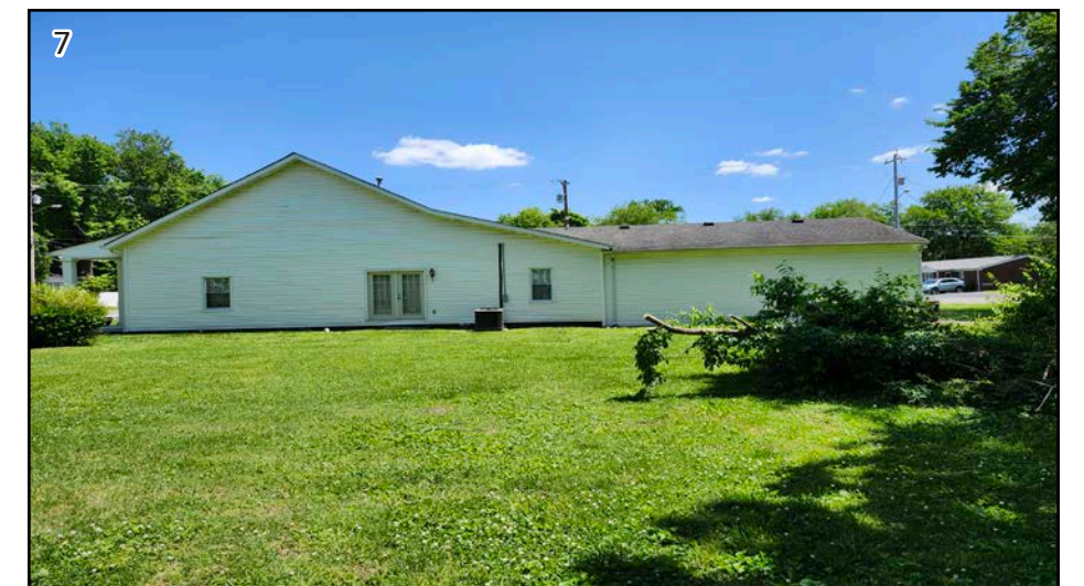
VIEW FROM SOUTHERN BOUNDARY LOOKING NORTH TOWARDS EAST VINE STREET
