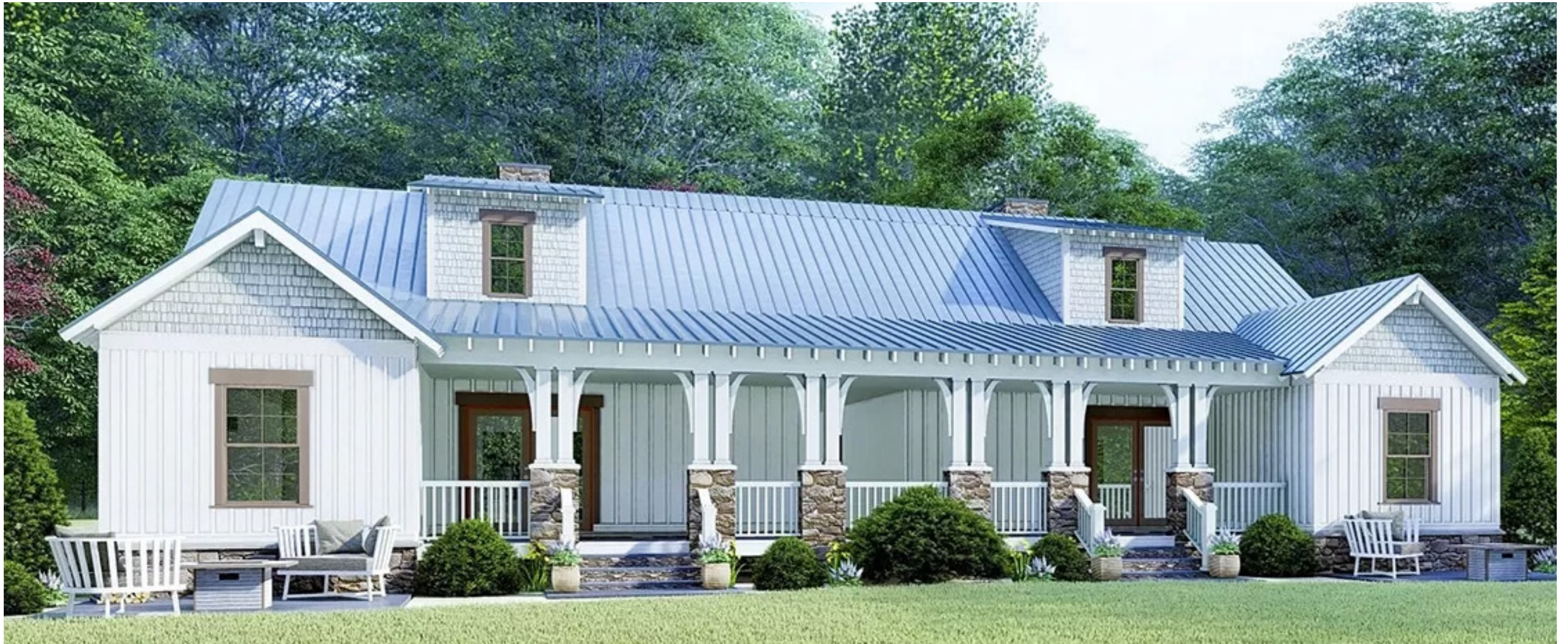
Rear elevation as seen from center courtyard
