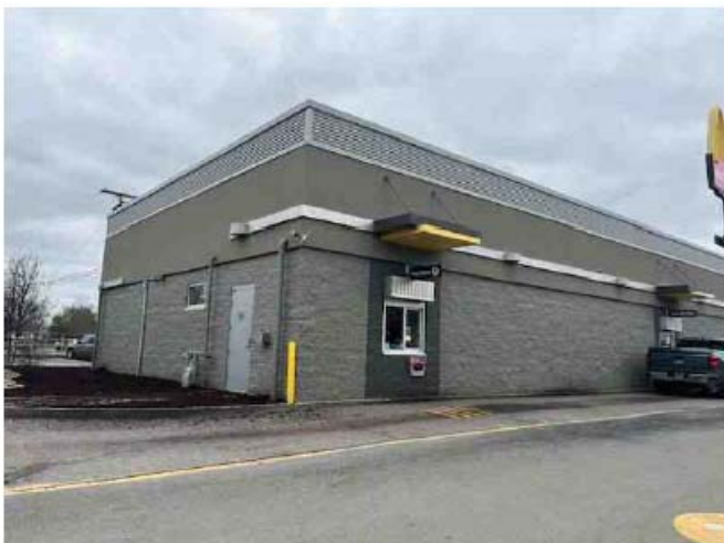
Rear/Side Structure 1 and view of Abandonment Easement Area (Easement F)
