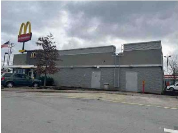
Side View Structure 1 and view of abandonment easement (Easement F)
