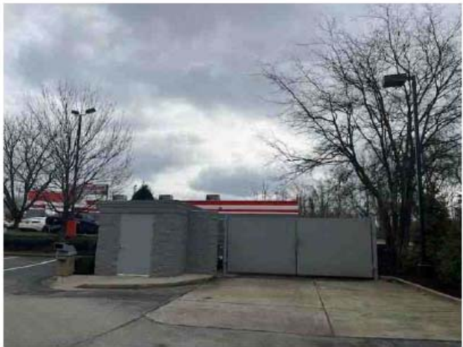
Storage and Dumpster Enclosure at SE Corner
