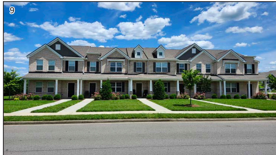
View of Neighboring Townhomes from Salem Creek Drive Looking East
