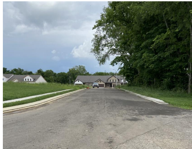
PHOTO 4: WESTRIDGE DRIVE @ WOODCREST DR LOOKING EAST
