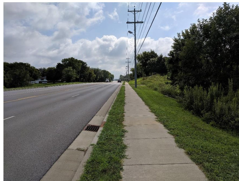
PHOTO 4: VETERANS PARKWAY CONNECTION LOOKING EAST
