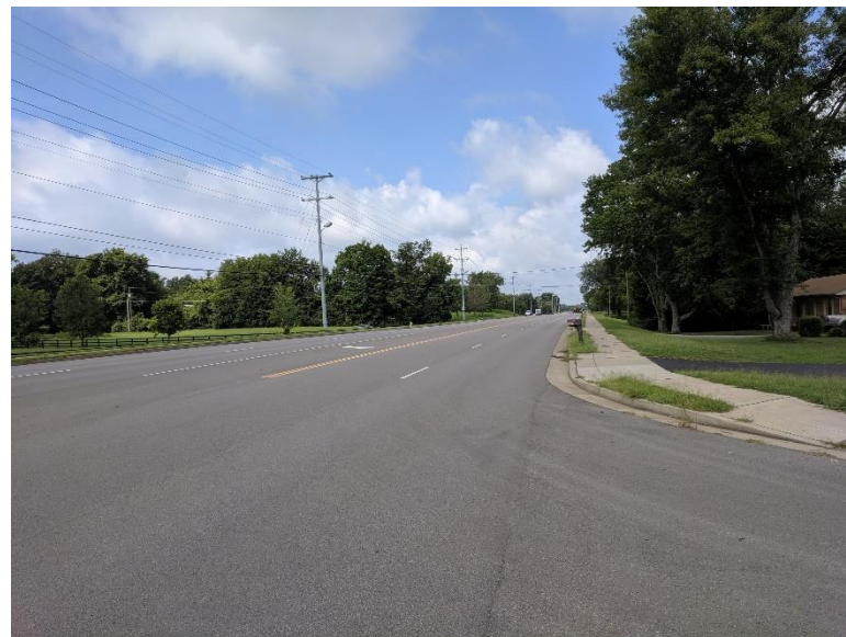
PHOTO 1: GREENVIEW DRIVE @ VETERANS PARKWAY LOOKING WEST
