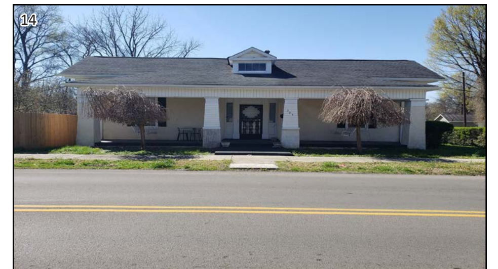
VIEW OF EXISTING FRONT ELEVATION ON ADJACENT PROPERTY
