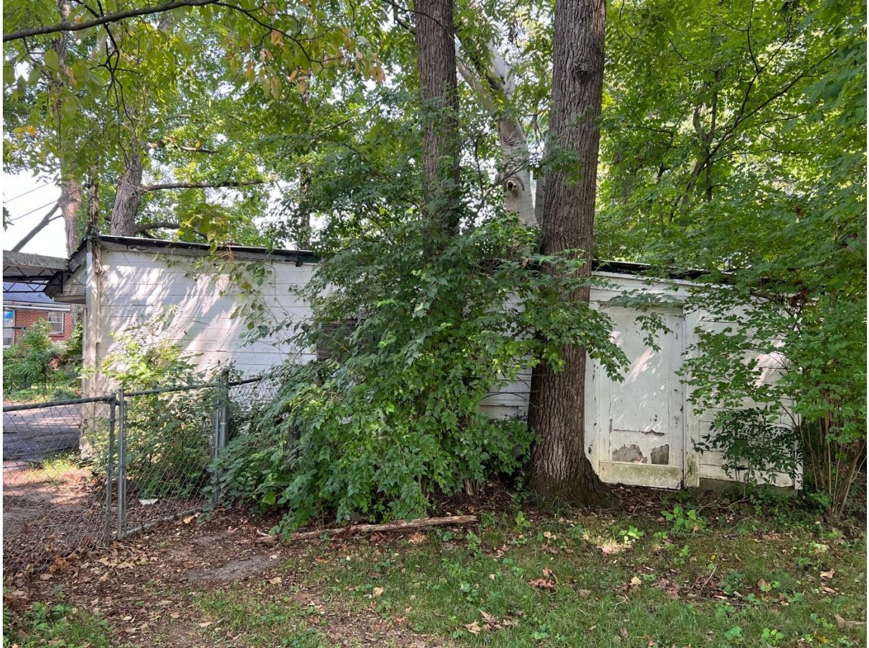
Side view of storage building. Walnut trees pictured to remain post-demo.
