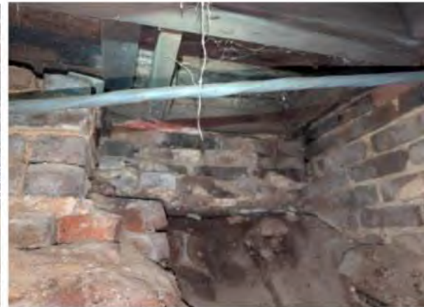
Failing brick wall
