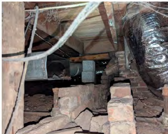
Failing brick, poor supports
