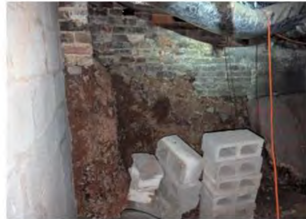
Erosion, failing brick foundation wall, no footing
