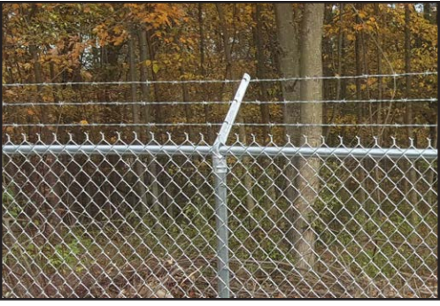
Example of Phase 1 Proposed Chain Link Security Fencing (±378 LF)
